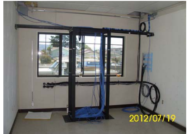
Rough in Cabling and Rack for MDF Room
