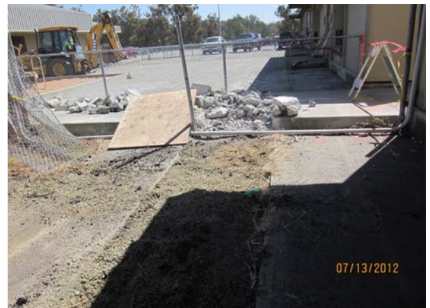
Trenching for Underground Utilities
