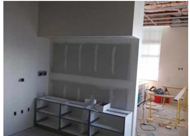
Construction of Sterilization Wall
