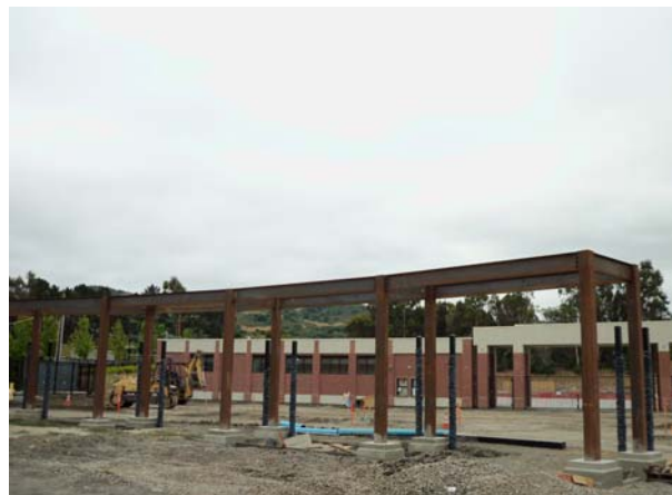
Building 14--Portico Steel Installation
