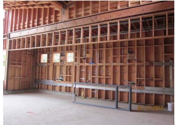
Classroom Interior Framing/ Rough-in Electrical
